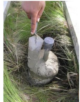
14. Place a 1.5 inch PVC pipe or 4 ft fiberglass rod near the SET point to aid locating it in the future. Check local conventions (NE: rod is to upland; NJ rod is to N)
