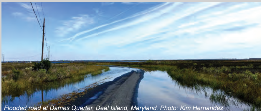
Flooded road at Dames Quarter, Deal Island, Maryland. Photo: Kim Hernandez
